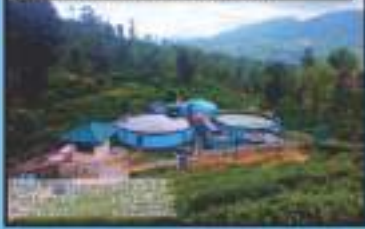
Bridwell Water Supply Scheme
