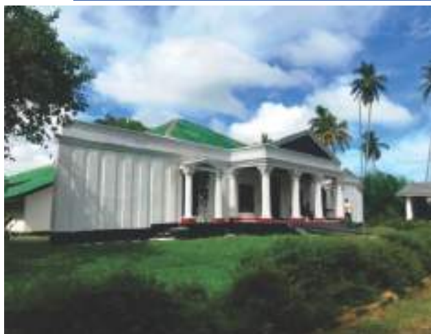
Renovation of Resource Centre-Galle Region
