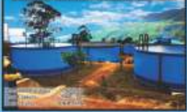
Fairburn Water Supply Scheme
