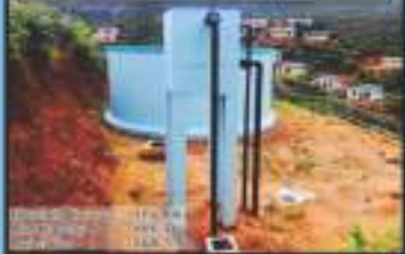
Lynsted Lower Water Supply Scheme
