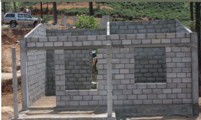
Nuwara Eliya Region - Diyagama West Estate
