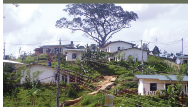
Kegalle Region - Atale Estate
