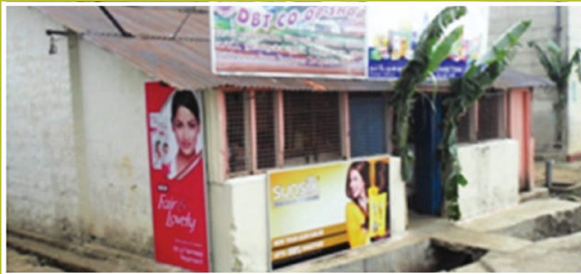
Refurbished EWHCS shops – Vellovo Estate and Dambetanna Estate
