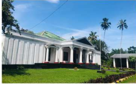
02 - Galle Regional Office
