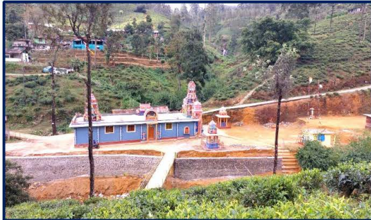
Kovil Retaining Wall- Diyagama East
