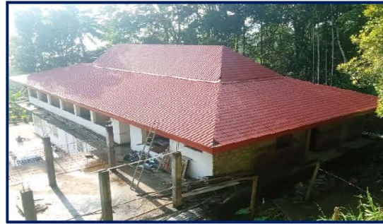
Rawanagoda Temple- Construction
