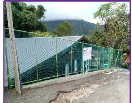
Retaining wall for COVID ward Dikoya Base Hospital
