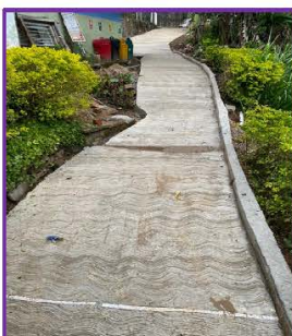
Foot Path & Drain Lindula Hospital
